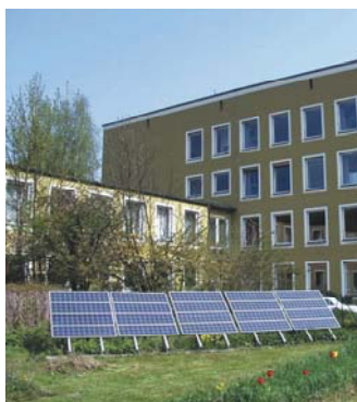
Figure 2: Sun at School - 1.1 kW PV system of a grammar school in Passau in the south of Germany
