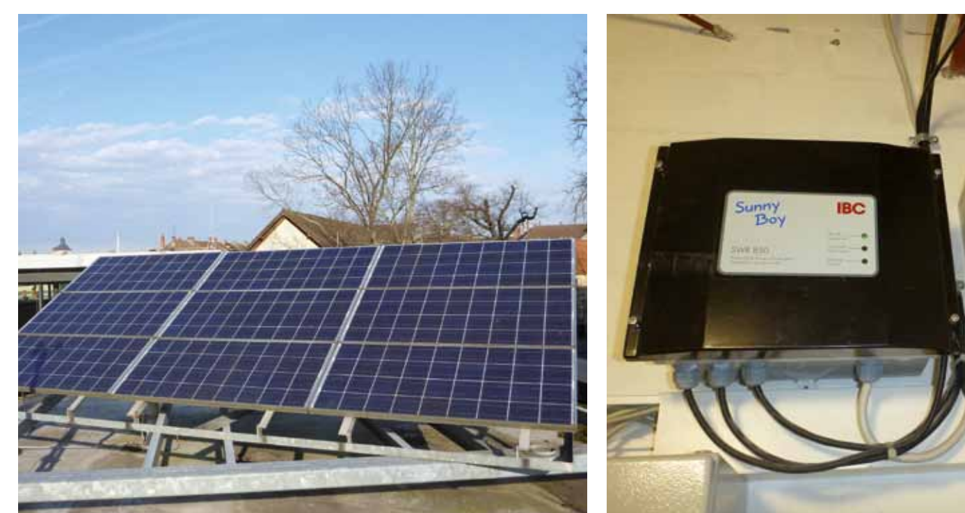
Fig. 3: SONNEonline PV system (9 x Kyocera KC120-1, inverter Sunny Boy SWR 850) of a grammar school in Braunschweig in the north of Germany
