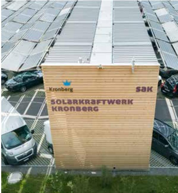
**Abb. 29:** Solarfaltdach HORIZON (429 kW) in Jakobsbad-Kronberg (dhp Technology AG)
